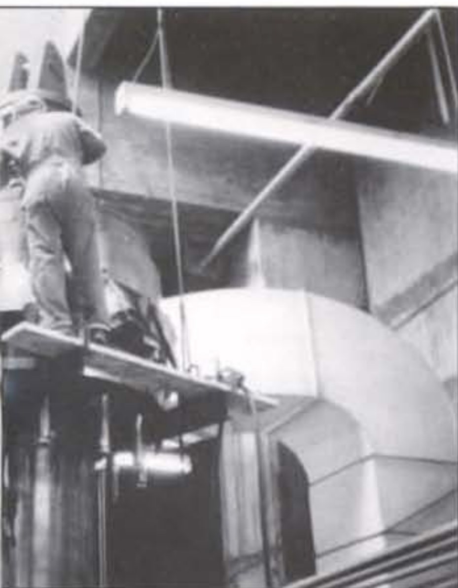
▲ Assembling a Thrust Runner to its Thrust Block and Shaft.
